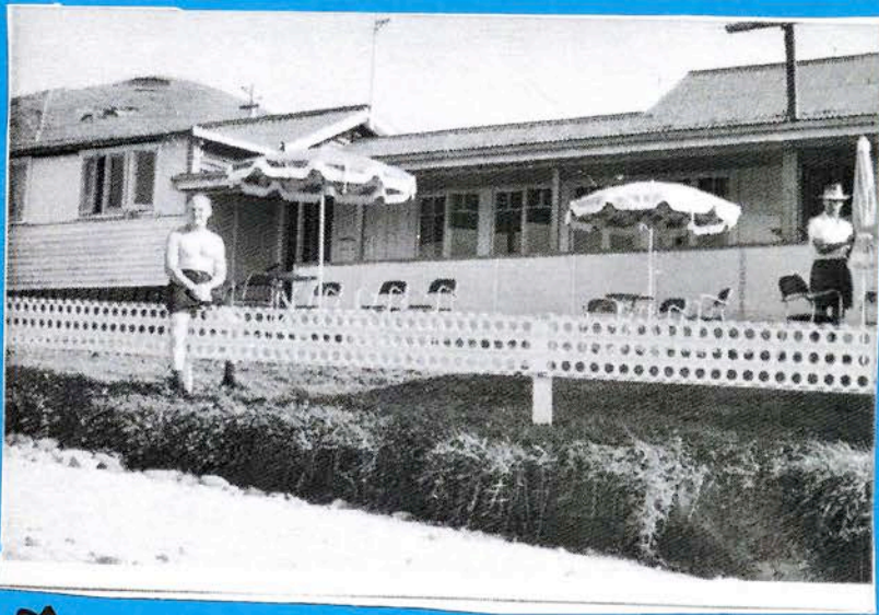
MARSDEN MATTING FENCE AT FRONT OF PARADISE.
