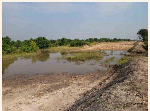
A pipeline route crossing a seasonal stream
